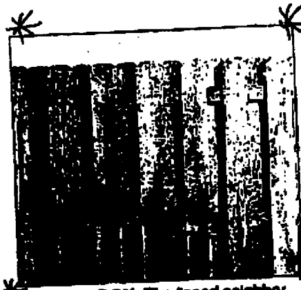
SHADOWBOX. The "good neighbor fence" has the same appearance on both sides.
