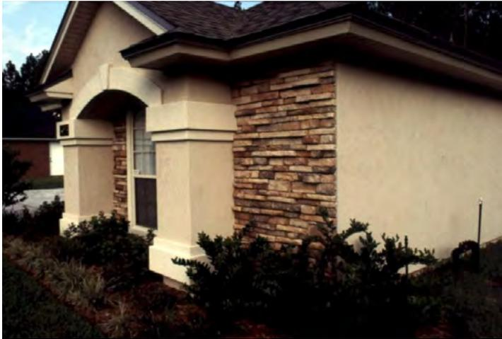
**Never change an exterior building material on an outside corner. Wrap materials at least 4'.**
